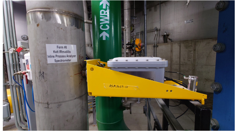
Photo: IRmadillo instrument installed in a recirculation line
