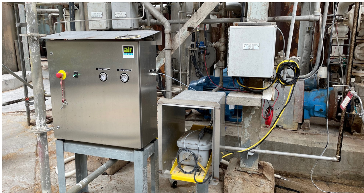
Photo: An IRmadillo process analyser installed in strong black liquor line, with accompanying compressed air dryer and filtration unit
